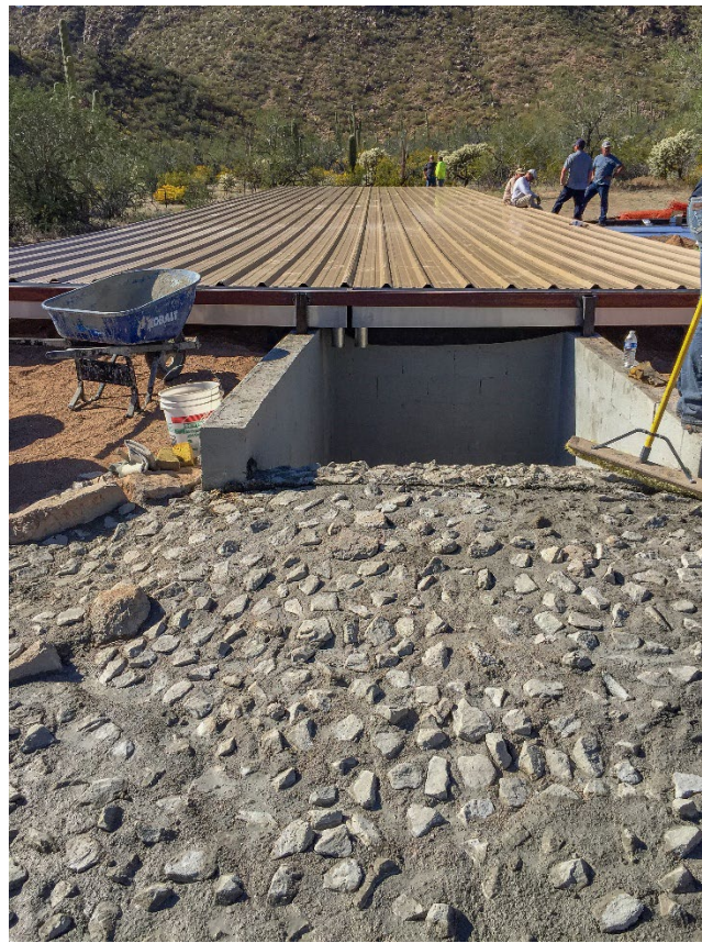
Water catchment rebuild in the western Silverbell Mountains. AZGFD photo by Rana Murphy
