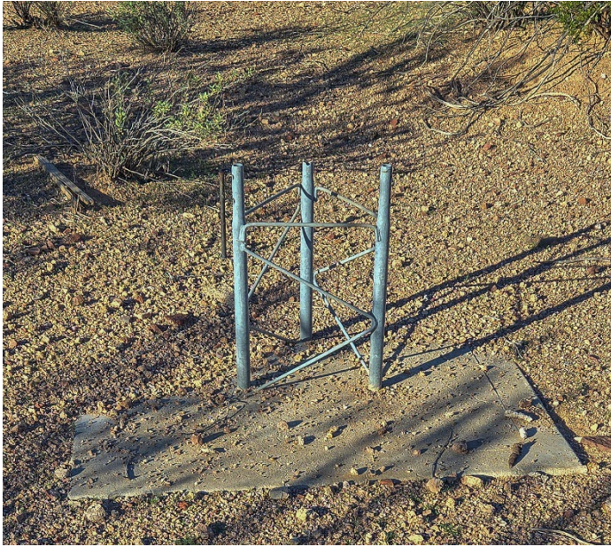
The base of the antenna tower used to transmit data from the meteorological station at the site to a receiver on Mount Lemmon.
